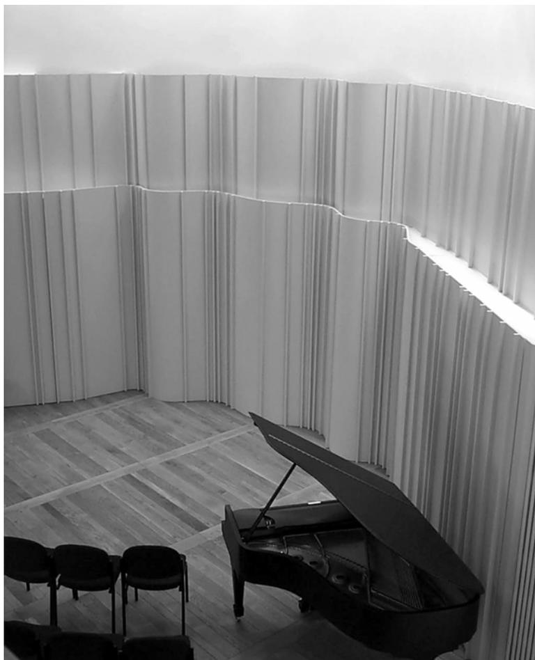
Figure 2.30 Optimized curved surface (OptiCurve™) in the Edwina Palmer Hall (photo courtesy of Arup Acoustics).
