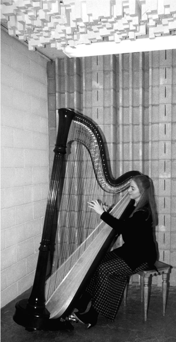
*Figure 2.14* A music practice room treated with diffusers (Skyline<sup>®</sup> on the ceiling [14] and DiffusorBlox<sup>®</sup> on rear wall [13]) and absorbers (after D'Antonio and Cox [1]).
