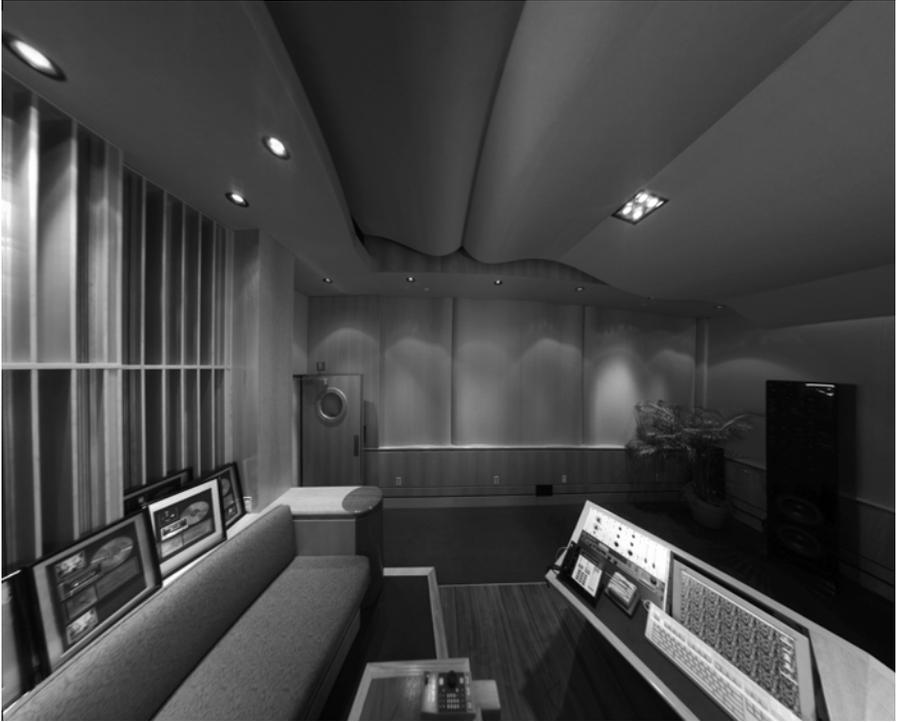
*Figure 11.5* A curved hybrid diffuser (Digiwave), applied to the ceiling and side walls of SonyM1, New York (photo by Paul Ellis of The M Network Ltd courtesy of Harris Grant Associates).
