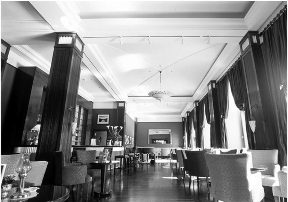
*Figure 1.1* Absorbent plaster ceiling applied to a restaurant (photo courtesy of BASWA acoustic, AG).
