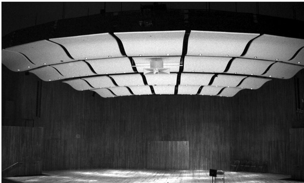
Figure 2.22 Overhead stage canopy at Kresge Auditorium, Boston, MA (Waveform™) (photo courtesy of RPG Diffusor Systems Inc.).
