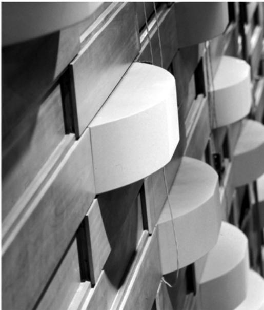
Figure 2.2 Application of optimized curved diffusers (OptiCurve™) in the Hummingbird Centre, Toronto (after D'Antonio and Cox [1]).
