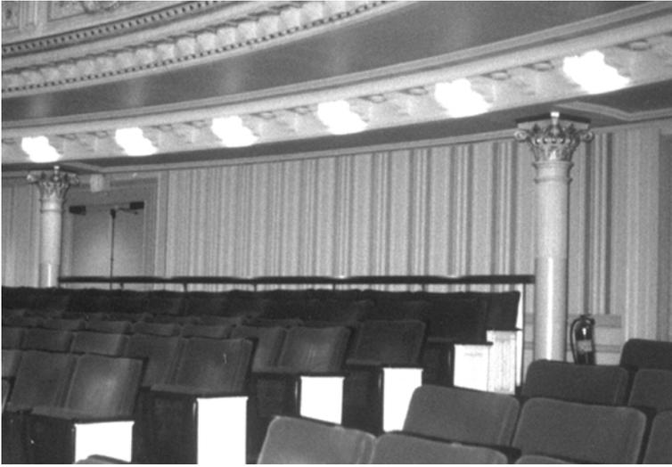
*Figure 2.1* Schroeder diffusers (QRDs<sup>®</sup>) applied to the rear wall of Carnegie hall to prevent echoes (after D’Antonio and Cox [2]).
